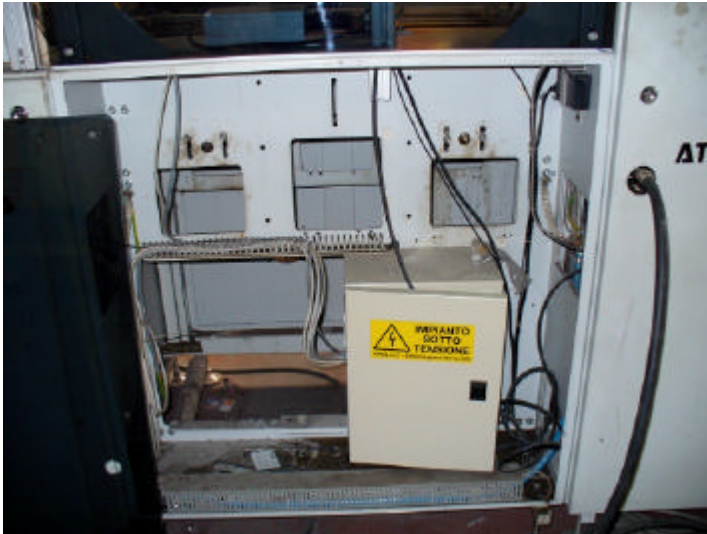
Example of insertion of the electrical panel inside Cart Line Module
